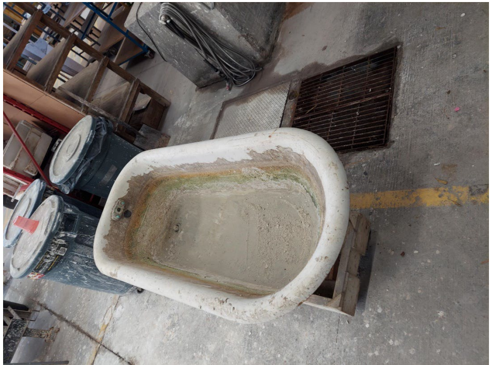
Photograph 8: Bathtub requiring stabilization.
