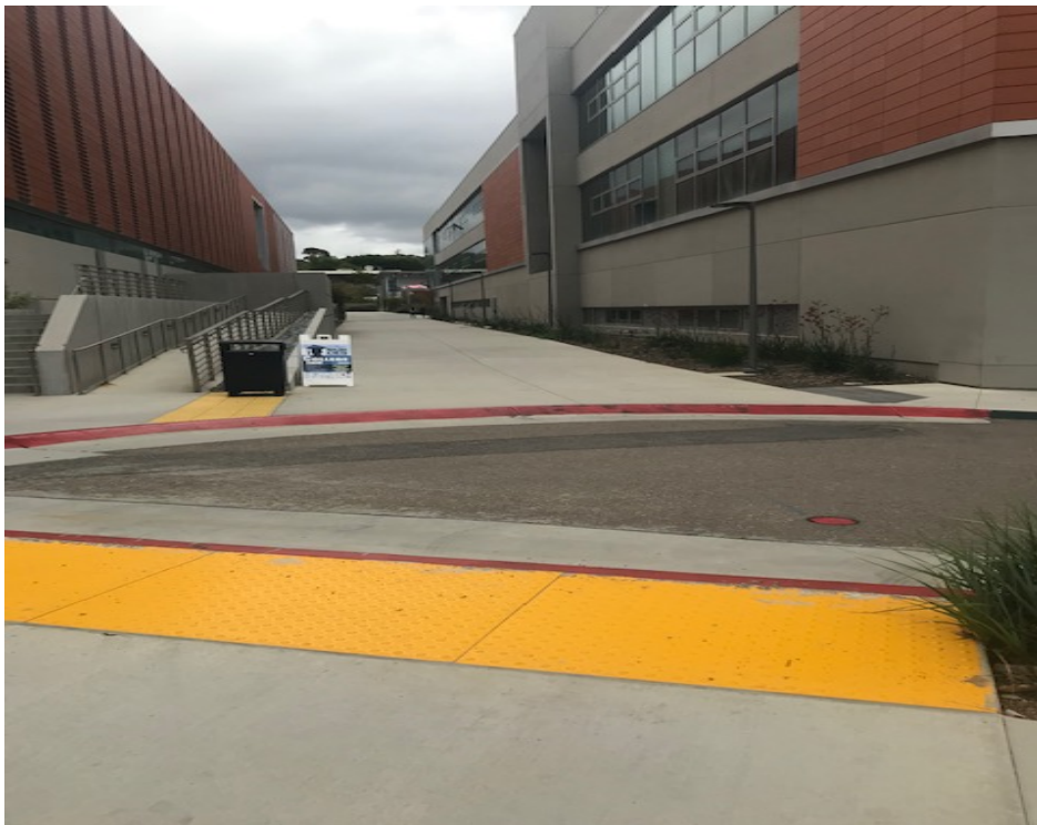
Walkway between H/MD- Bldg. facing Comet Circle
