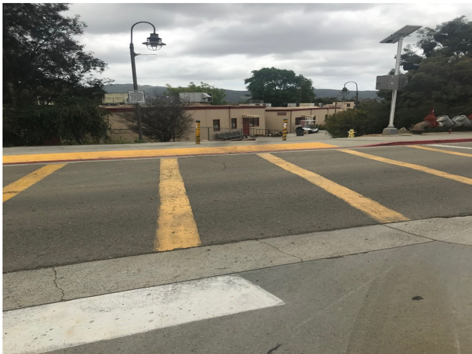
Walkway adjacent to RS-Bldg.
