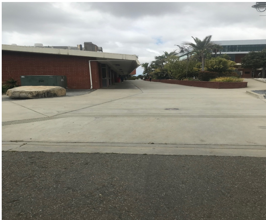
Walkway by F-Bldg.
