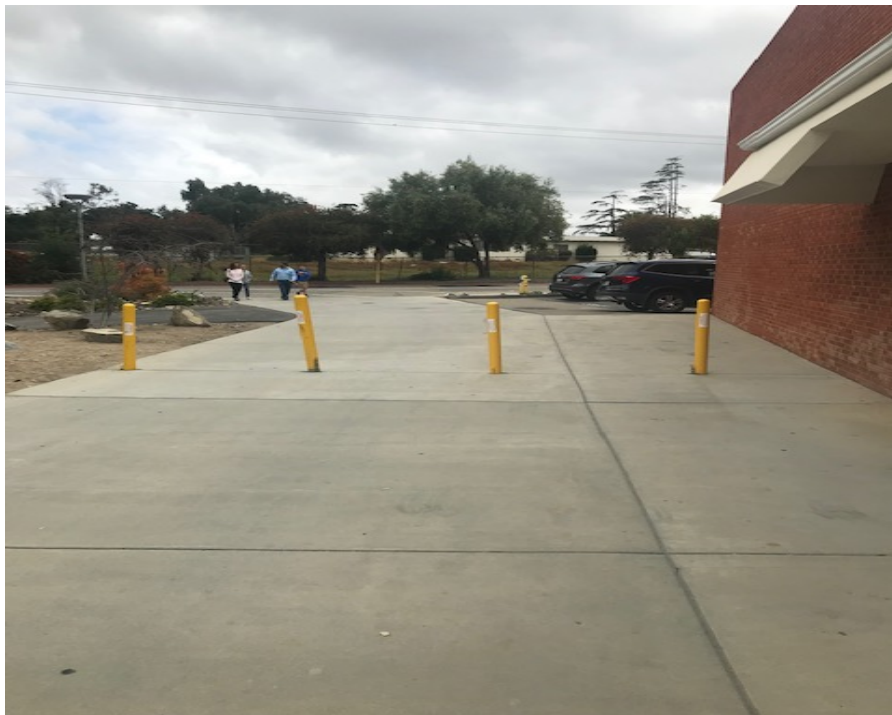
Walkway between PAC/D-Bldg.
