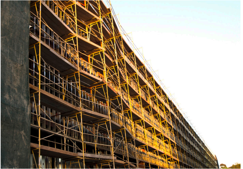
February 2013 Humanities Building Construction
