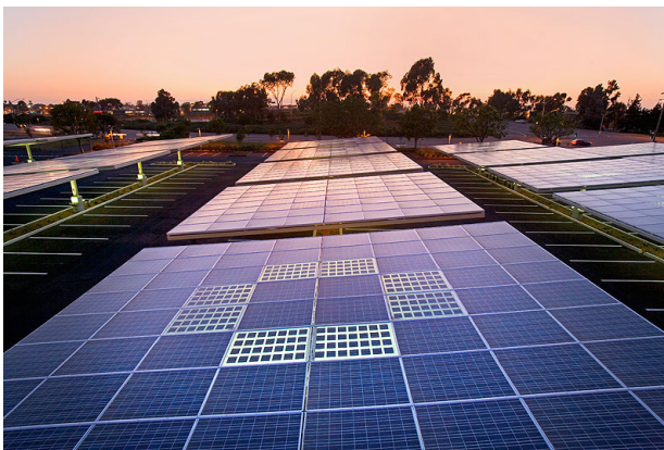
Solar PV array with integrated lighting
