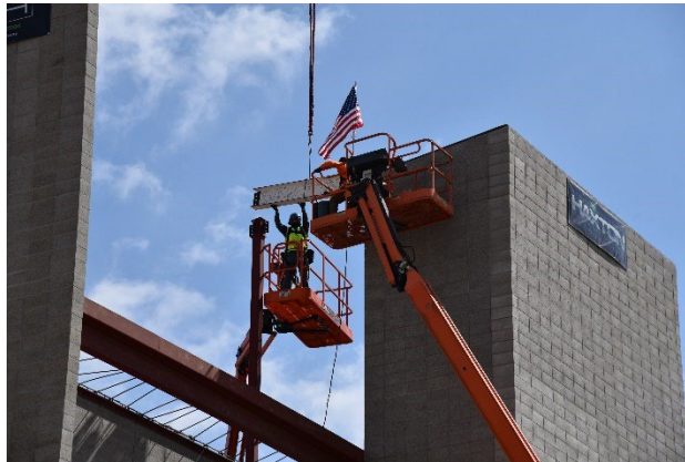
Placement of the beam at the top of the football stadium press box
