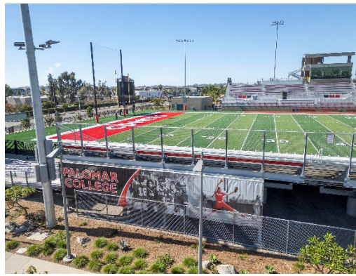
The visitor side bleachers windscreen project at the football stadium.
