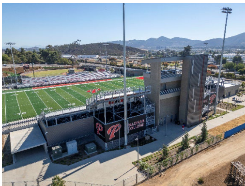
The home side bleachers windscreen project at the football stadium.
