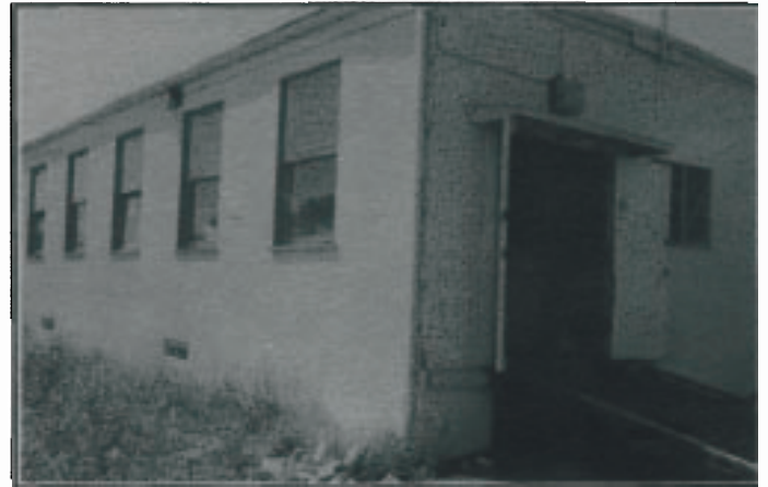
One of a few of the earliest buildings of 1950 on Palomar College campus, still in use as a storage facility.
