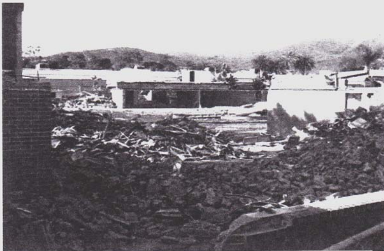
Rubble from Construction Site
