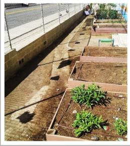
Needs Improvement: Gardens on pavement close to storm drain swale; dirt and irrigation water entering swale
