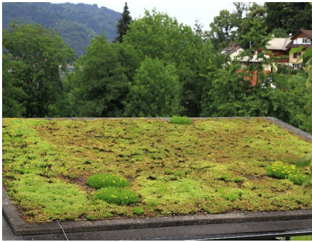
Green roofs provide an opportunity to utilize traditionally unused spaces for stormwater management.
