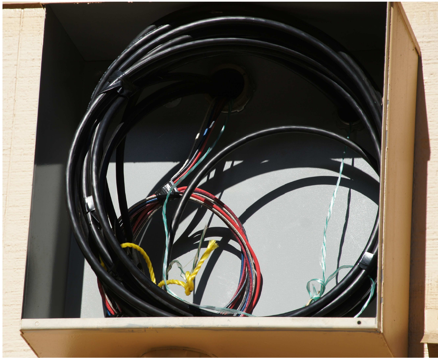
2 EXISTING PULLBOX FOR FIBER AND TELEPHONE
