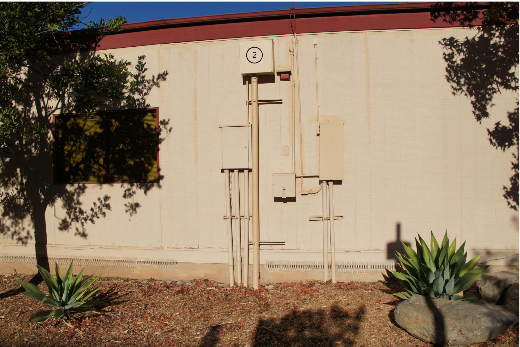
3 EXISTING PULLBOXES, TIME CLOCK AND POWER PANEL
