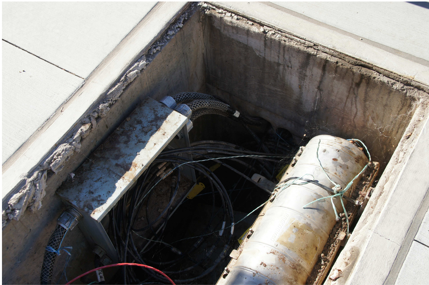
1 EXISTING FIBER TUBE AND TELEPHONE POINT OF CONNECTION
