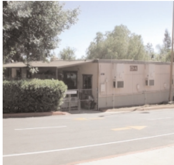
Image 7.41 One of the existing CDC temporary buildings along the road.
