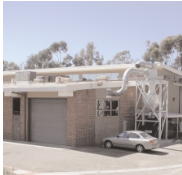
Image 4.4 T Building East Entry
