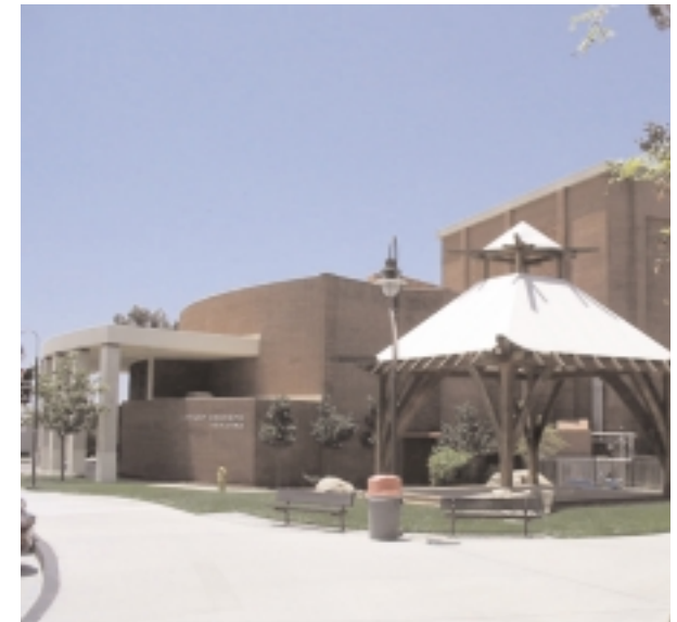
Image 4.5 Theatre East Facade
