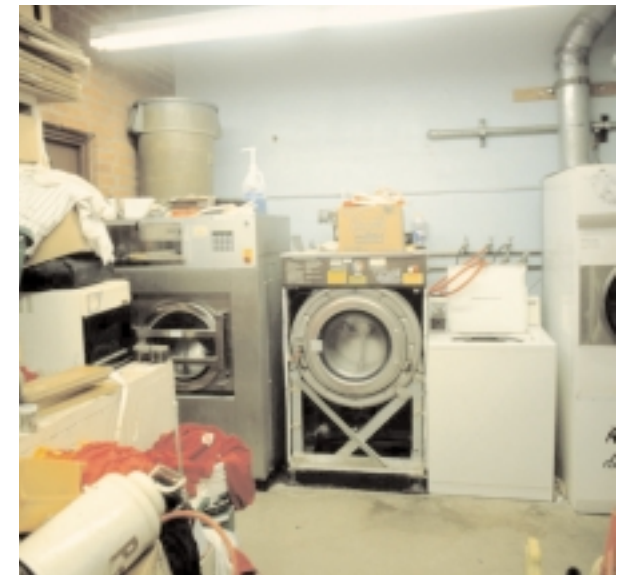
Image 7.76 M-Men's Locker Room Laundry Room
