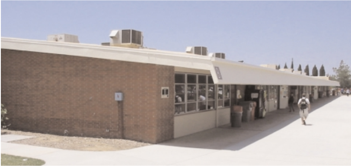
Image 4.2 Building B Northeast Corner
